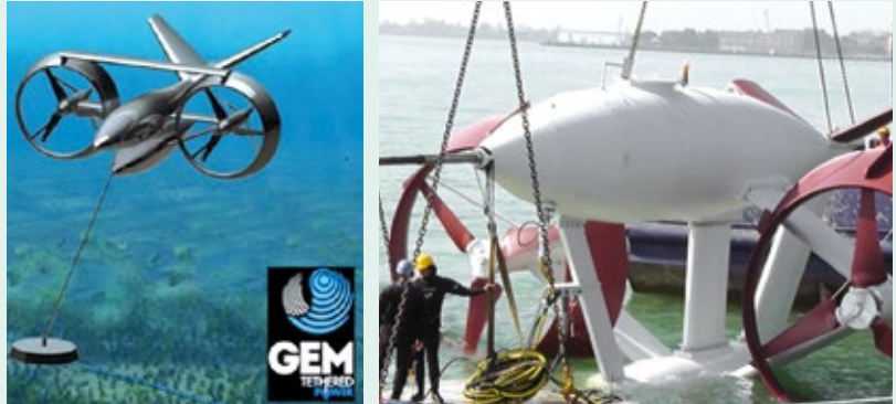
3D representation of GEM project (left) and installation of 100 kW prototype (right). Courtesy: Seapower
