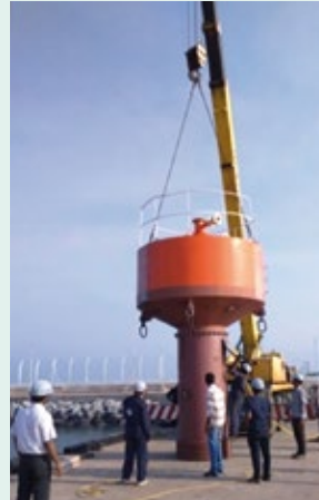
The floating OWC system at port prior to its deployment (left) and the system deployed in position (right)
