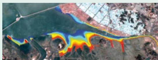
Aerial view of construction of Sihwa TPP (top) and restored tidal flat after operation of Sihwa TPP (down)
