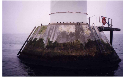
Concrete foundation (Vindeby)
