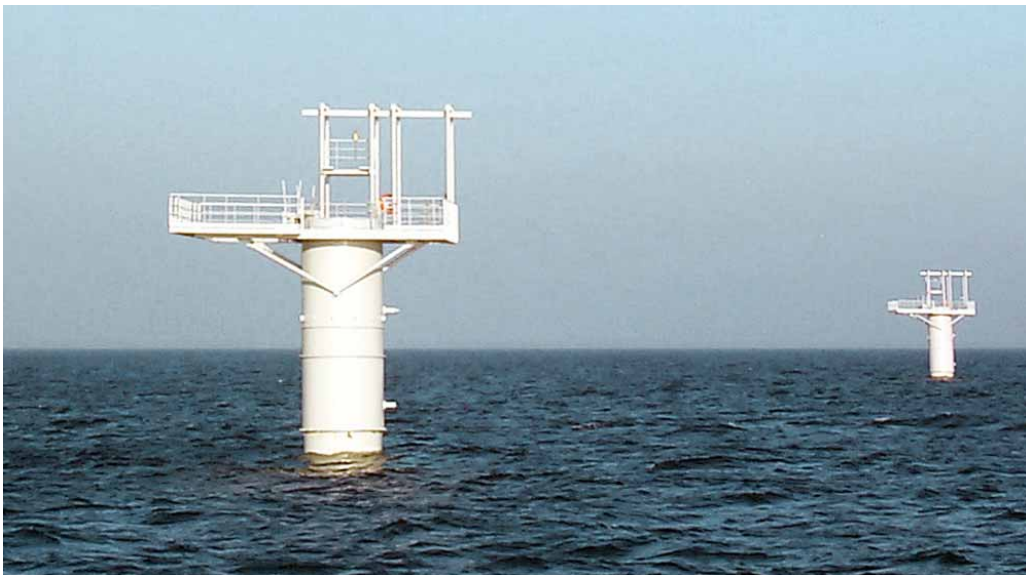
“Monopile” type-foundation
