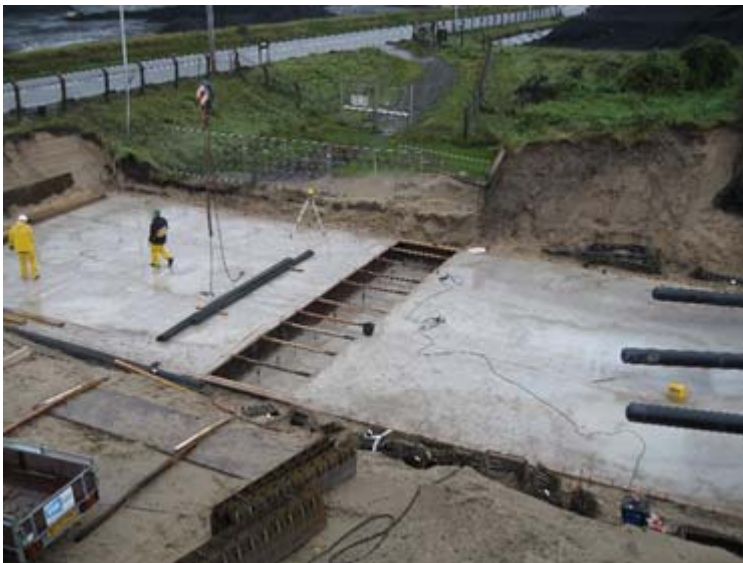
Substation floor and 3 pipes to conduct wind farm cables.
