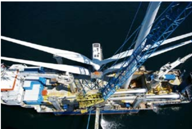
Sea Energy with two nacelle assemblies, seen from a just installed tower
