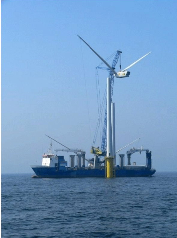
Nacelle installation with the Sea Energy
