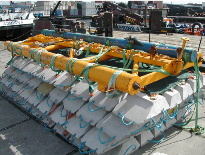
Photo: Mattress used for cable crossing separation
