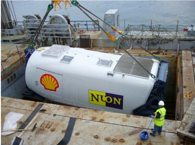
Nacelle transport by vessel.
