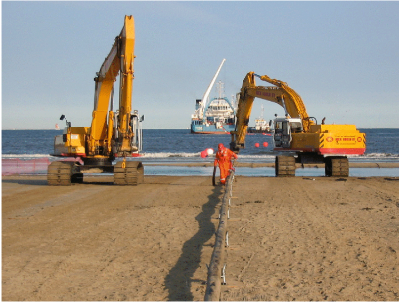
Cable lay vessel in front of shore and cable pull on beach.
