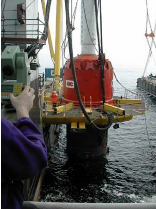
Monopile in piling frame with hydraulic hammer on top.
