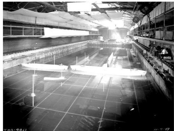
Figure 9. Navy's 1st Flap Wavemaker in the Experimental Model Basin (1913).
