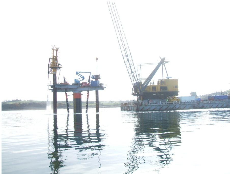
Figure 3-1 Photograph of pin pile drilling operations during the installation of the SeaGen tidal turbine device, Strangford Lough, Northern Ireland.
