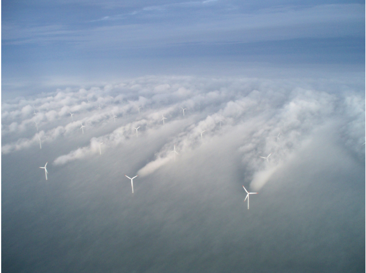
Figure 11. Horns Rev I wind farm (Source: Vattenfall, Photo by Christian Steiness )
