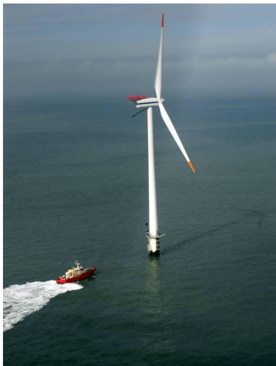
Figure 4-7. Maintenance boat in the Horns Rev I wind farm.
