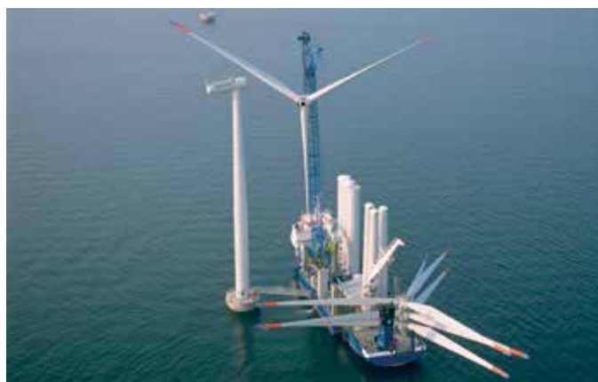
Marine wind turbine under construction off the coast of Denmark.
