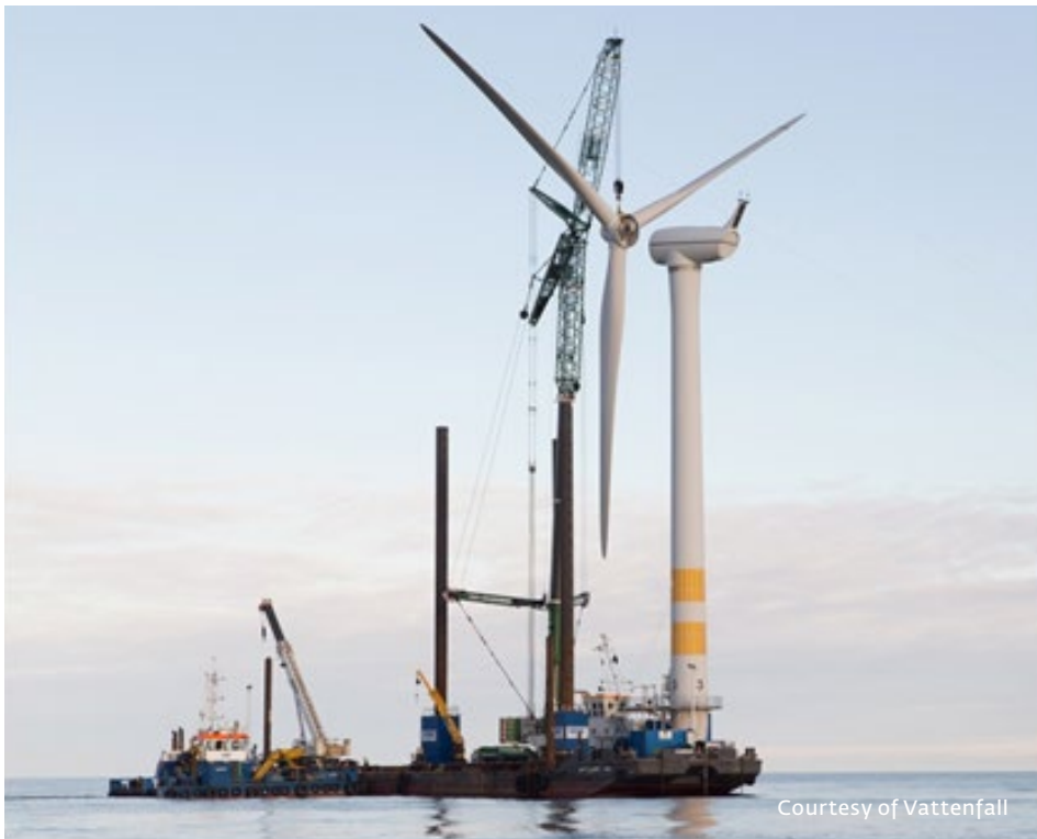
Figure 4 Decommissioning the Yttre Stengrund wind farm in February 2016.
