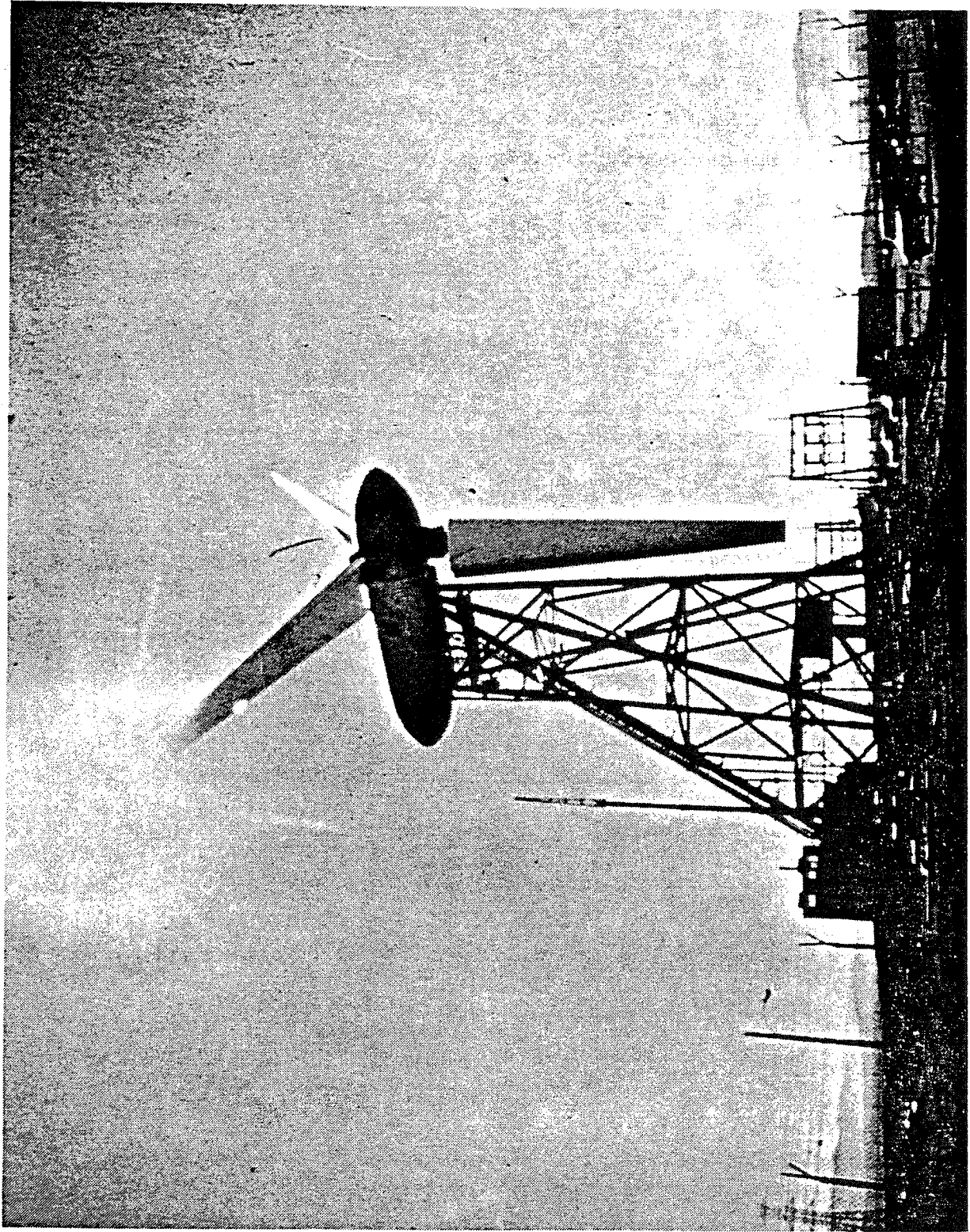
Figure 27. Bendix wind turbine constructed in 1980 near the Devers substation (maximum height = 58.7 m, rotor diameter = 50.3 m, rotor speed = 23 rpm). Study site 2 is located just east of this turbine (Figure 3).
