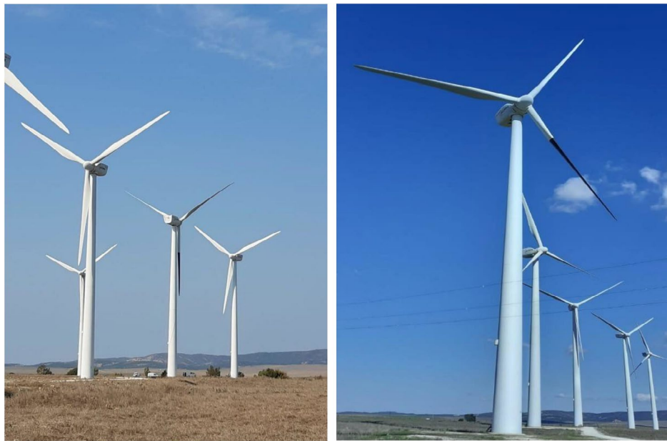
FIGURE 2 | Wind turbines at the El Ruedo wind farm with a blade painted black as a visual cue to birds to reduce collision fatalities.
