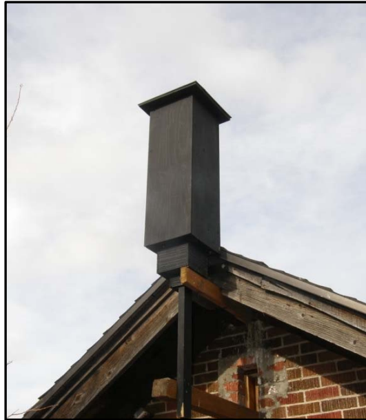
Rocket box bat house on eave with good solar exposure – Bryce Maxell
