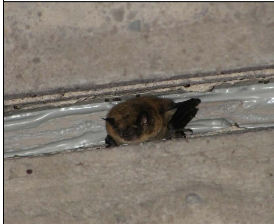
Big Brown Bat in highway expansion joint crevice – Bryce Maxell
