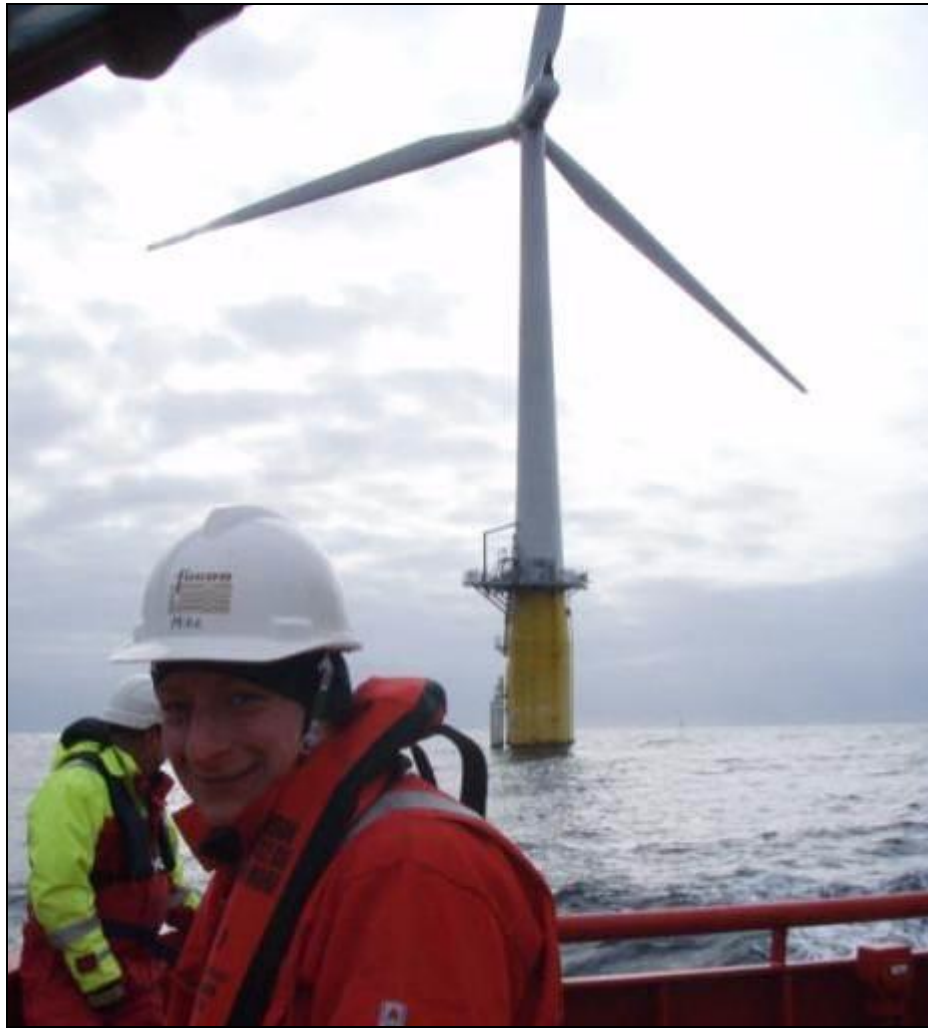
Figure 2: HYWIND floating wind turbine, 28 March 2011.
