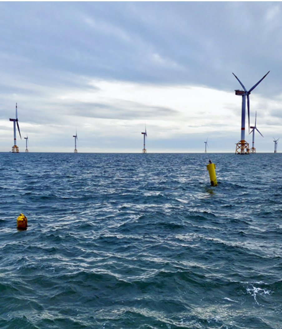
Offshore Belwind windpark (© Gust Lesage)
