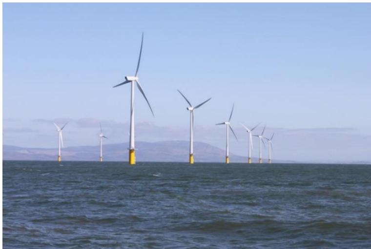
Figure 10: Robin Rigg OWF. Source: Arup
