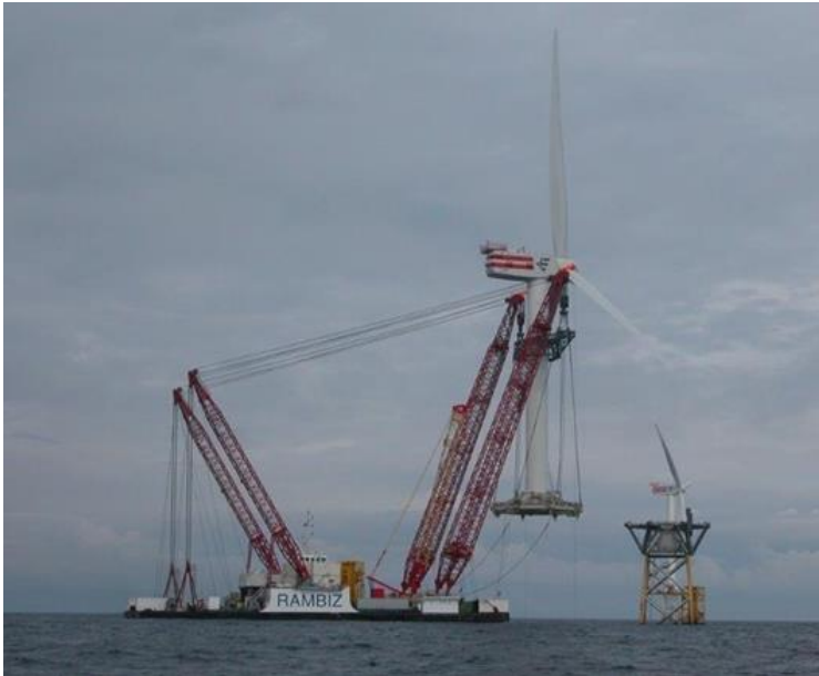
Figure 11: Installation of the complete Beatrice Demonstration WTGs. Source: Repsol Sinopec (35)
