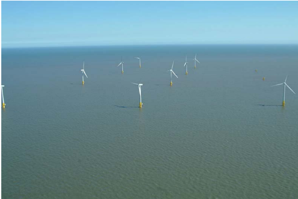
Figure 4 E.ON UK's Scroby Sand Wind Farm during Construction
