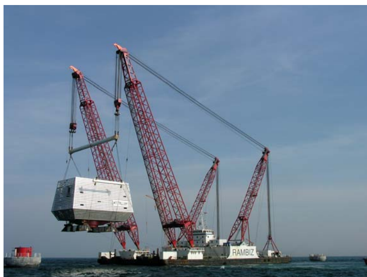
Figure 6 Installation of Offshore substation at Nysted Offshore Wind Farm
