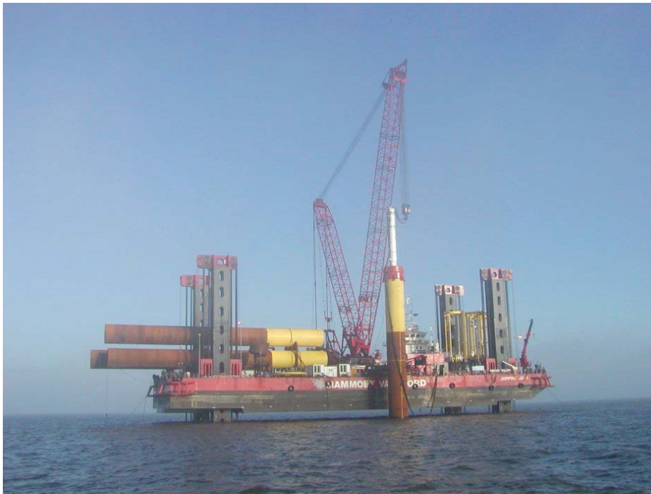
Figure 5 Monopile Installation at E.ON UK's Scroby Sands Wind Farm
