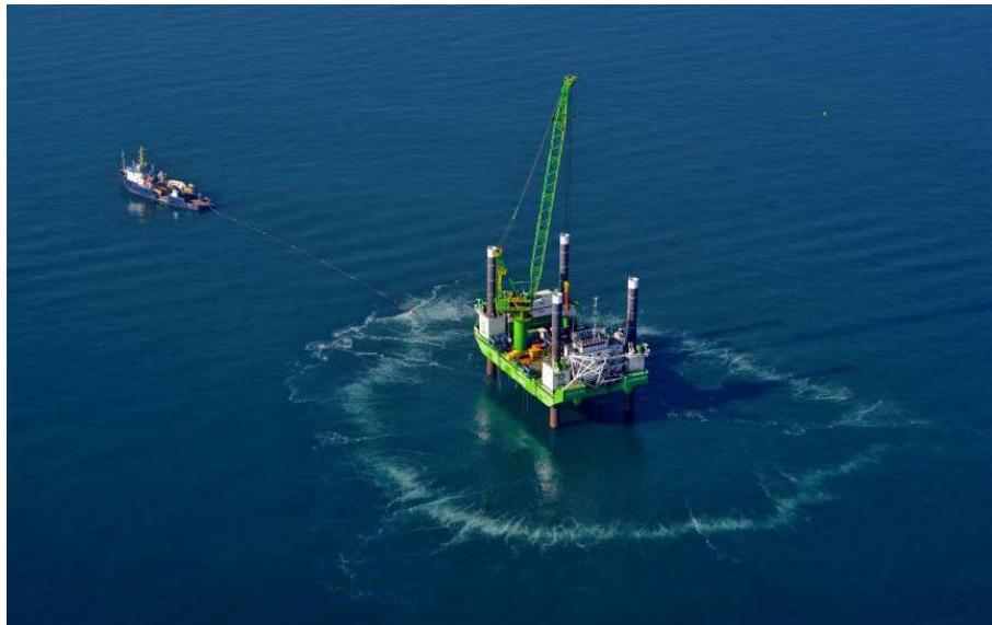
Figure 6: Application of a BBC by Hydrotechnik Lübeck at the OWF Borkum West II (photo: Trianel GmbH/Lang )
