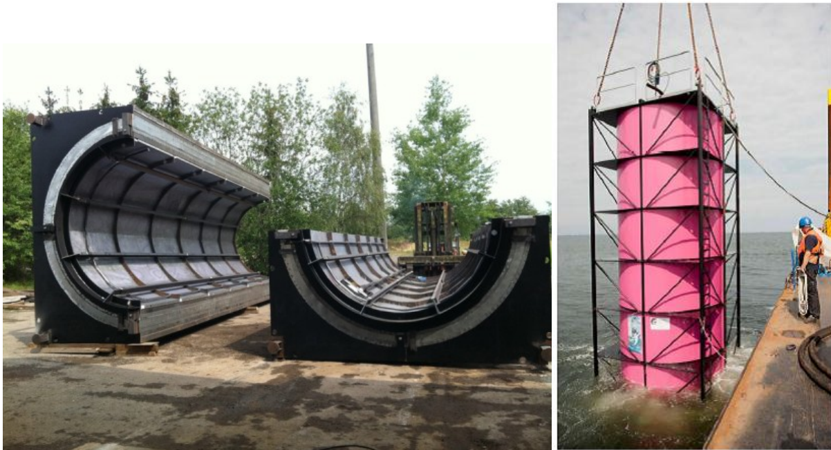
Figure 18: BEKA Shell by Weyres Offshore : Left: Half-shells opened (source: http://www.veyres-offshore.de/ ). Right: During the installation in the ESRa project (source: WILKE et al. 2012, photo: PATRICE KUNTE)
