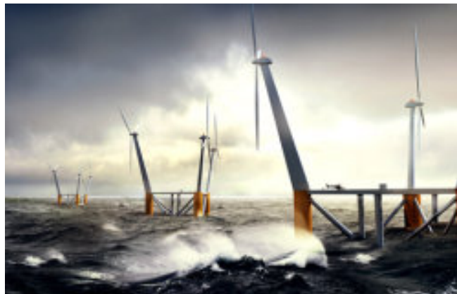
Figure 58: WINDSEA concept of two upwind and one downwind operating wind turbines on the same floating foundation, a freely rotating semi-submersible (source: WINDSEA AS)
