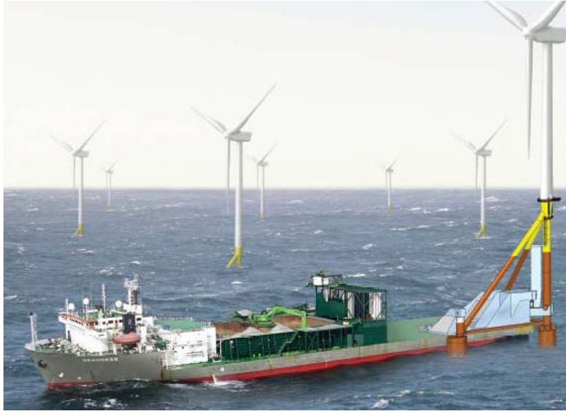
Figure 63: Asymmetric three-legged jacket design with bucket foundations (source: SPT Offshore , Woerden, The Netherlands)
