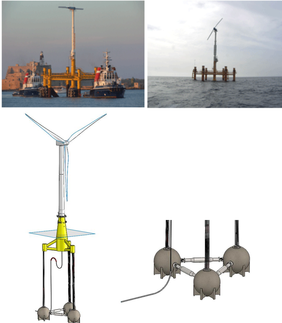
Figure 55: Wind turbine on Blue H Submerged Deepwater Platform SDP. Top: first prototype tested offshore from 2007 to 2009 (source: Blue H , Oosterhout, The Netherlands, www.bluehgroup.com ). Bottom: concept of a 5 MW prototype with submergible gravity based anchor weights (Quelle: Nico C. F. BOLLEMAN, Blue H Engineering BV , The Netherlands)
