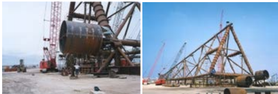
Figure 67: Jacket for offshore oil platform with suction buckets (source: SPT Offshore , Woerden, The Netherlands, www.suctionpile.com )
