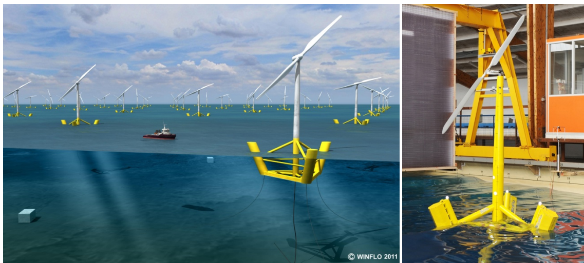
Figure 60: A two-blade wind turbine on a semi-submersible construction is realized in the WINFLO concept. Left: an artist's view of a WINFLO windfarm, right: model test in a wave tank in October 2011 (Copyright: WINFLO 2011)
