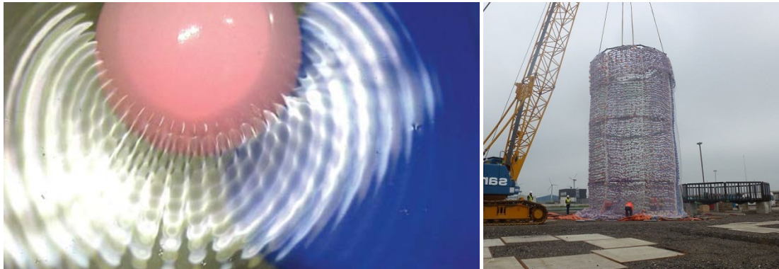
Figure 30: Scattering and absorption tests with HSD balloons in a wave flume (left) und preparations for practical application of an HSD net ( \varnothing 9m, height 28 m, weight of the complete system 17 t) at the OWF London Array (right) (sources: ELMER et al. 2011, 2012)
