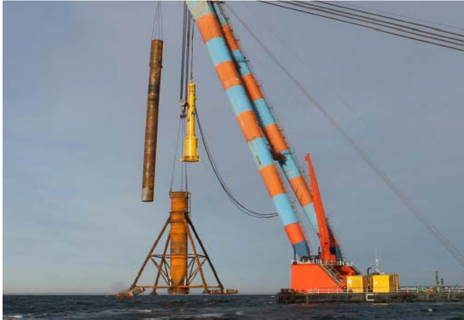
Figure 25: Cofferdam by Lo-Noise/SeaReenergy during the test at Aarhus Bight (source: THOMSEN 2012)
