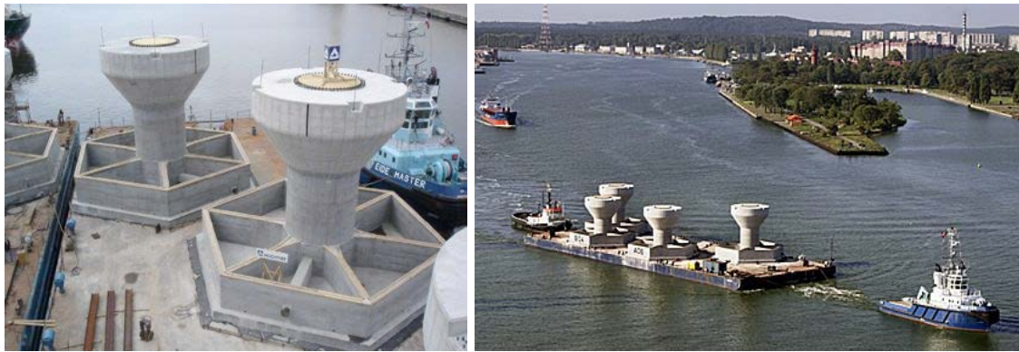
Figure 50: Gravity base foundations of the OWF Lillgrund (source: left VATTENFALL 2008, right: FREISEN 2010)
