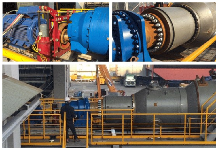
Figure 9. Dynamo test pictures for PMSG and Drivetrain of 200 kW TEC.
