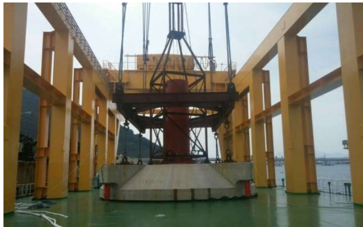
Figure 8. The caisson-type gravity-based support structure.
