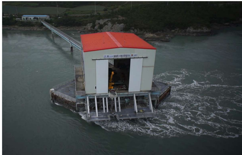
Figure 7. A photo of the Uldolmok Tidal Current Power Pilot Plant.
