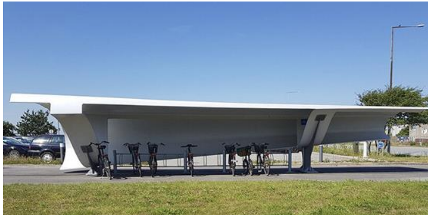
Figure 25. This repurposed-blade bike shelter was installed by the wind turbine manufacturer Siemens Gamesa in collaboration with the Re-Wind Network. It is located in the port of Aalborg, Denmark.
