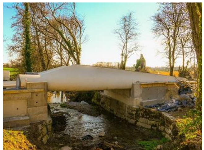
Figures 3 & 4: BladeBridge's pedestrian bridge on the Midleton-Youghal Greenway, Cork, Ireland
