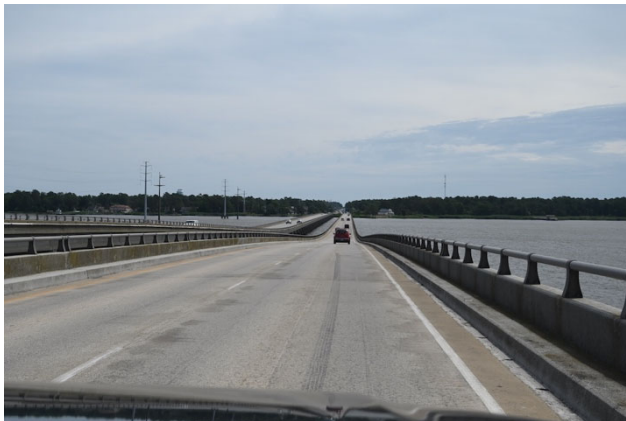
Route 158 bridge over Currituck Sound toward Southern Shores.
