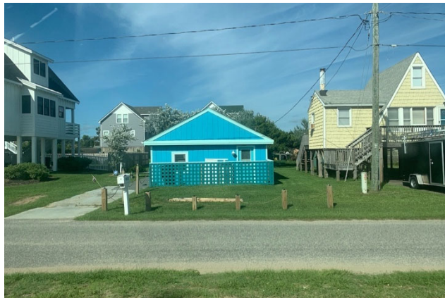
A few single-story homes remain on the Outer Banks. Most homes are raised to avoid storm surges.
