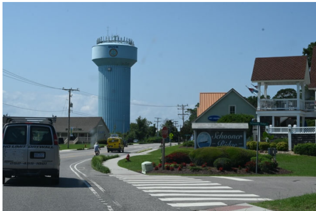
Water tower with co-located communications equipment, Duck.
