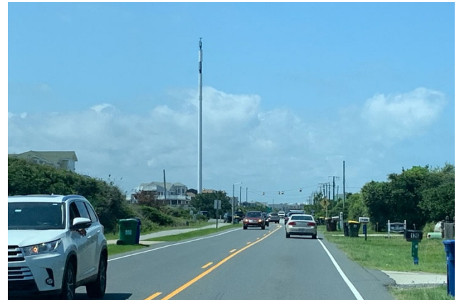
Contemporary monopole transmission tower near Route 12 in Southern Shores.
