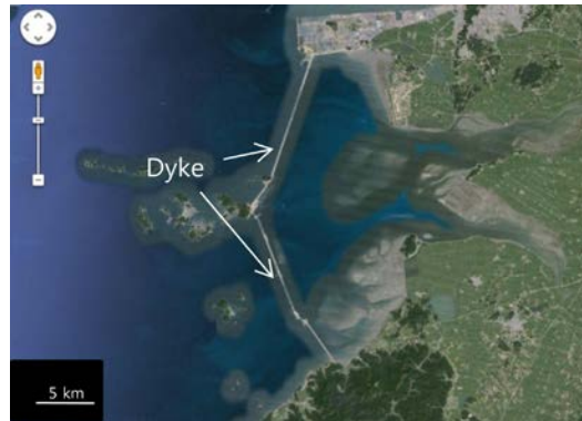
Fig. 3 Saemangeum reclamation located in western South Korea (Scale: 5 km, photo by Google).
