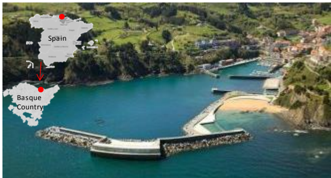
Figure 1: Mutriku OWC plant
