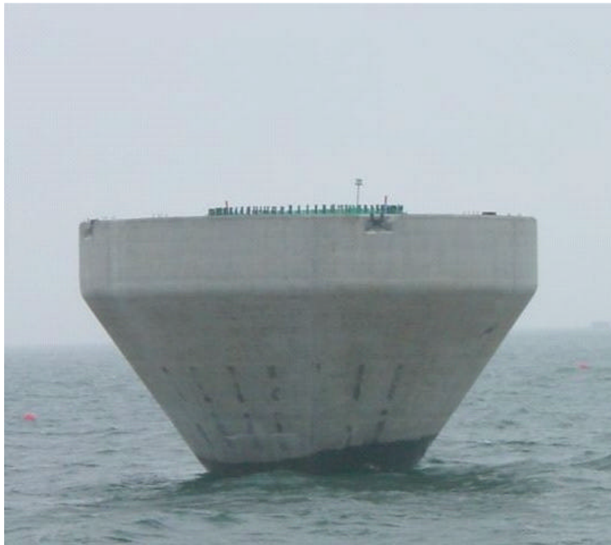
Figure 6.3. Picture of one of the turbine foundations put in position in the wind farm area.
