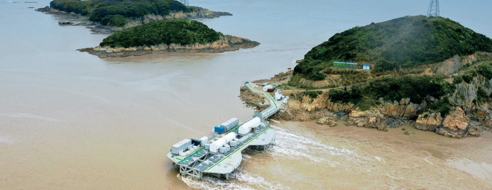
LHD Tidal Current Energy Demonstration project, Xiushan Island, China Courtesy: LHD
