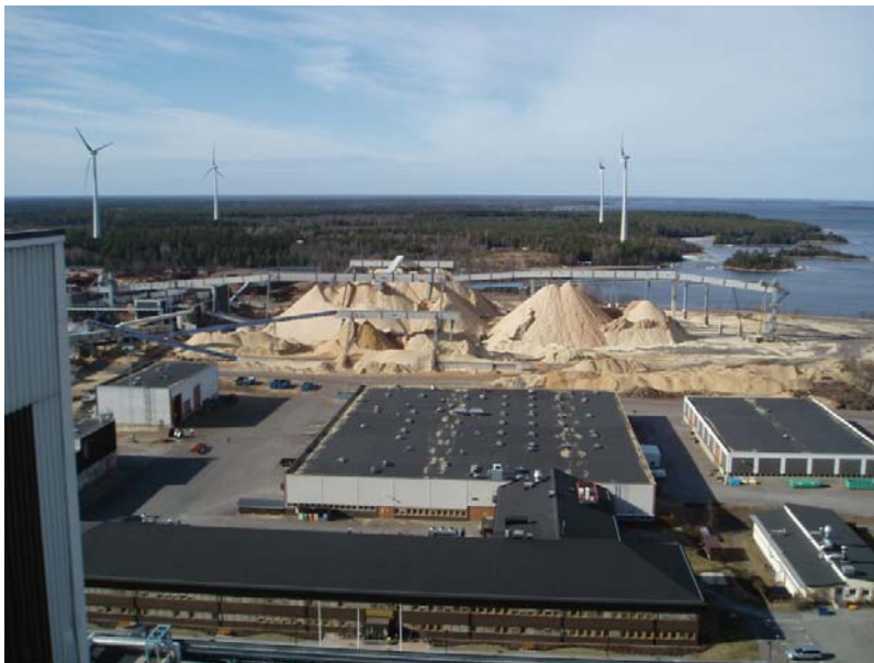
Figure 4.2. Wind power in an industrial landscape (Photo: Annika Andersson)
