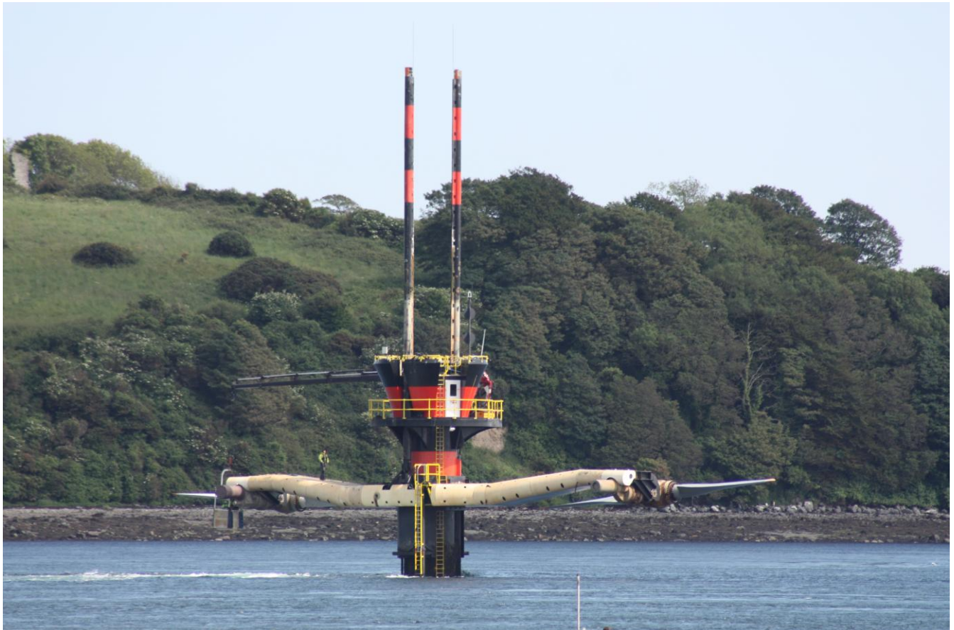
Figure 1 The SeaGen tidal turbine, a commercial-scale horizontal-axis TCC deployed in Strangford Lough, Northern Ireland [18].
