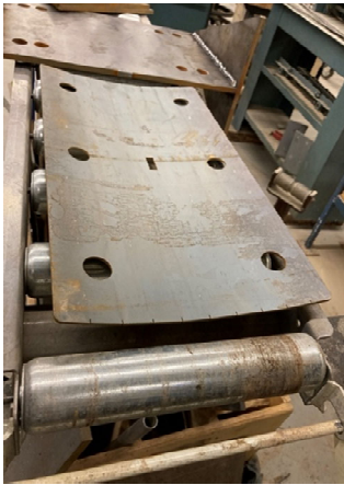
Figure 10: Steel is formed to fit blade curvature
