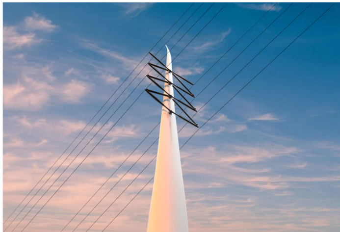
Figure 1: Detail of BladePole with Braced Line Post Hardware
