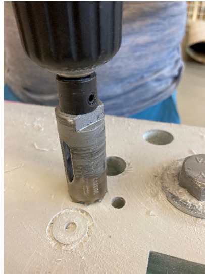
Figure 13: Drilling of hardware holes with diamond saw
