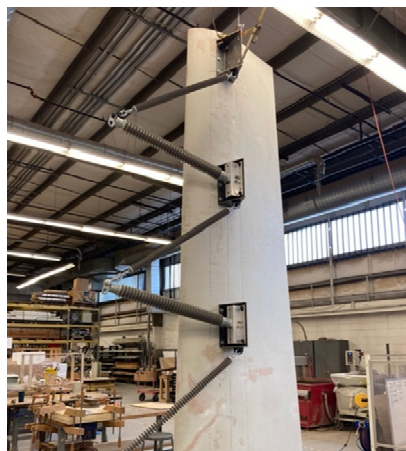
Figure 15: UC and Braced Line Post hardware is completely installed and blade is erected in the lab awaiting a full-scale structural test
