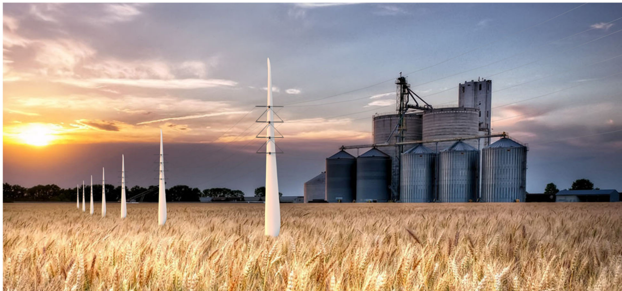
Figure 2: BladePole as a series of straight run Tangent Poles in a double circuit 230 KV transmission line
