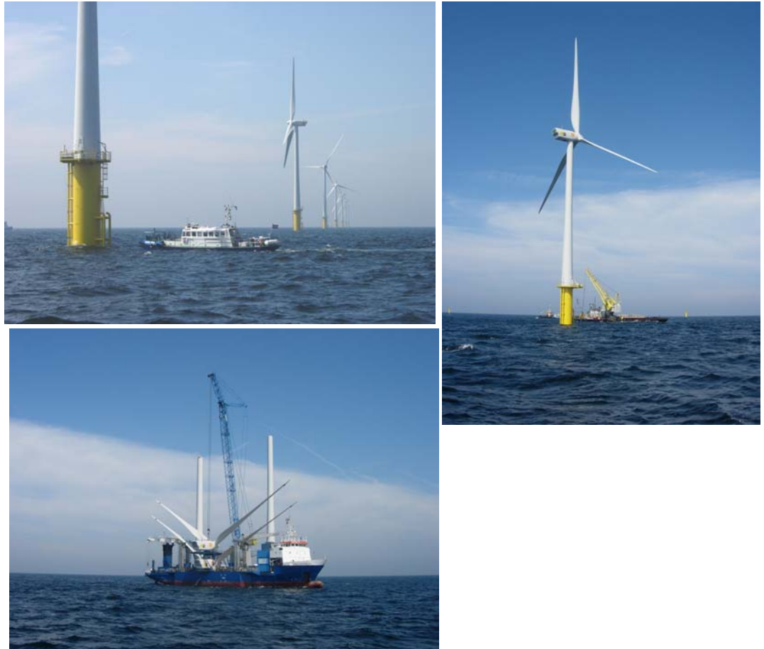
Figure 3 The building of the Off-Shore Wind farm Egmond aan Zee (OWEZ) in the Dutch coastal zone 8 - 18 km of the coast of Egmond aan Zee with 36 wind turbines with a total capacity of 108 MW.
