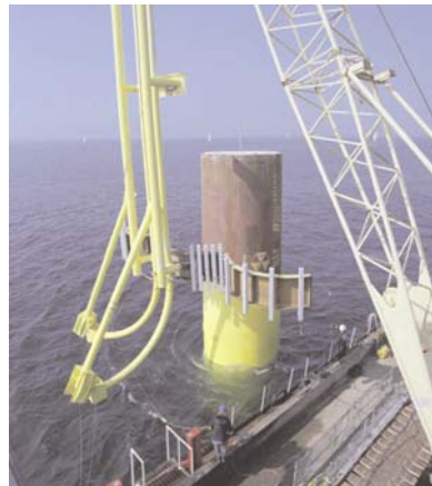
Figure 15. Installation of J-tubes
