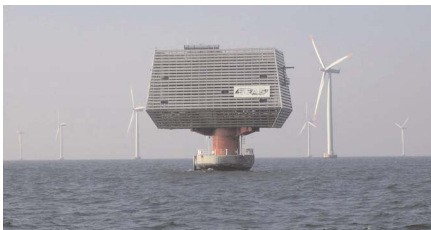
Figure 16. An example of an offshore substation
