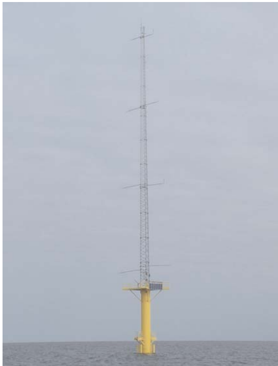
Figure 17. Met-mast installed at the eastern boundary of Gwynt y Môr
