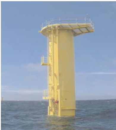
Figure 14. Installed transition piece
