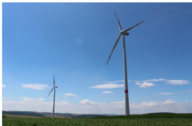
Fig. 9 The main visible components of a wind turbine (Foto: taken from Friedrich-Wilhelm Raiffeisen Wind Farm Streu & Saale by the author)
