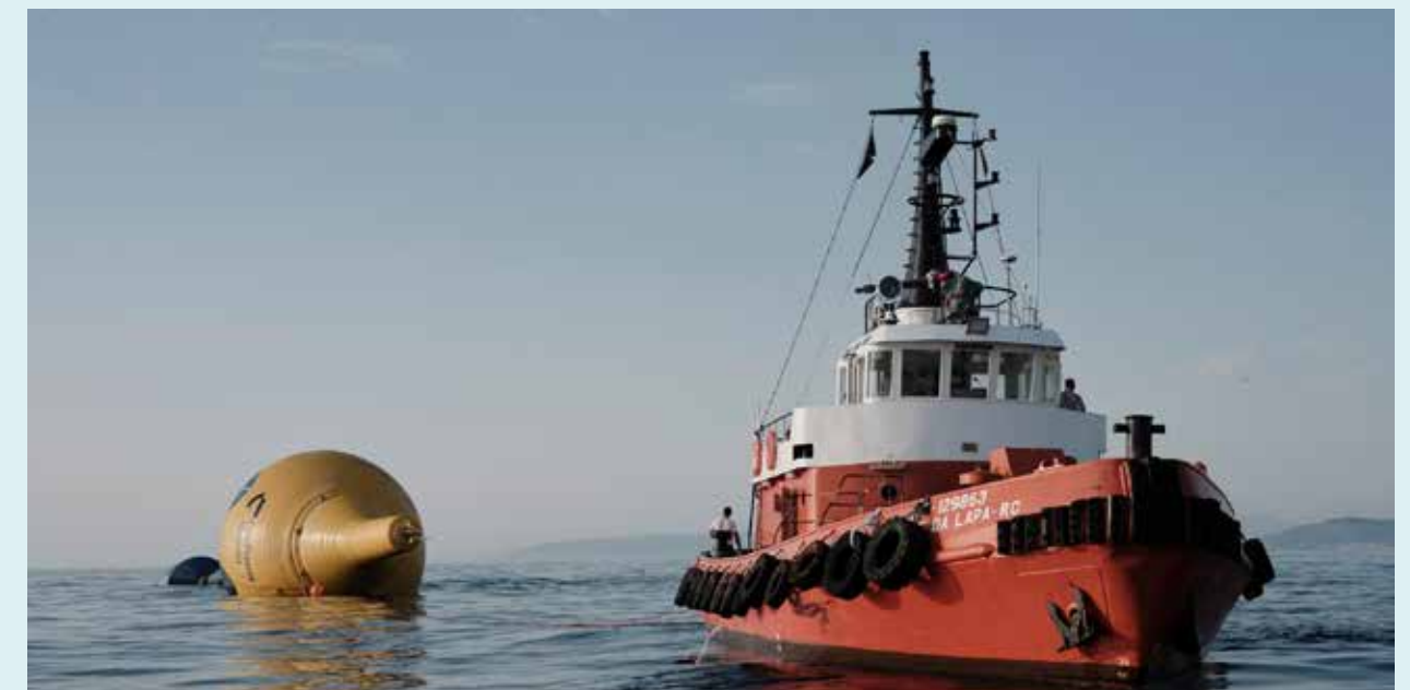
CorPower C4 device towed out during deployment (Credit: CorPower Ocean)
