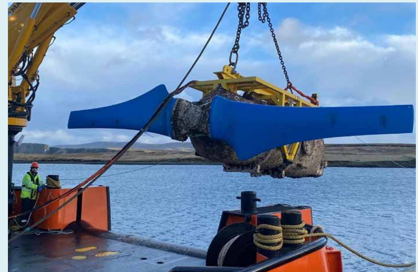
Nova Innovation completing tidal turbine maintenance (Credit: Nova Innovation)
