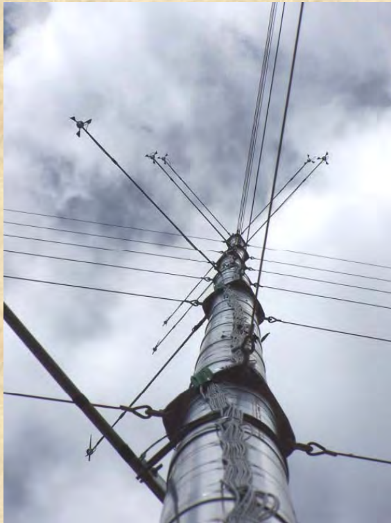
Typical Meteorological "MET" Tower
