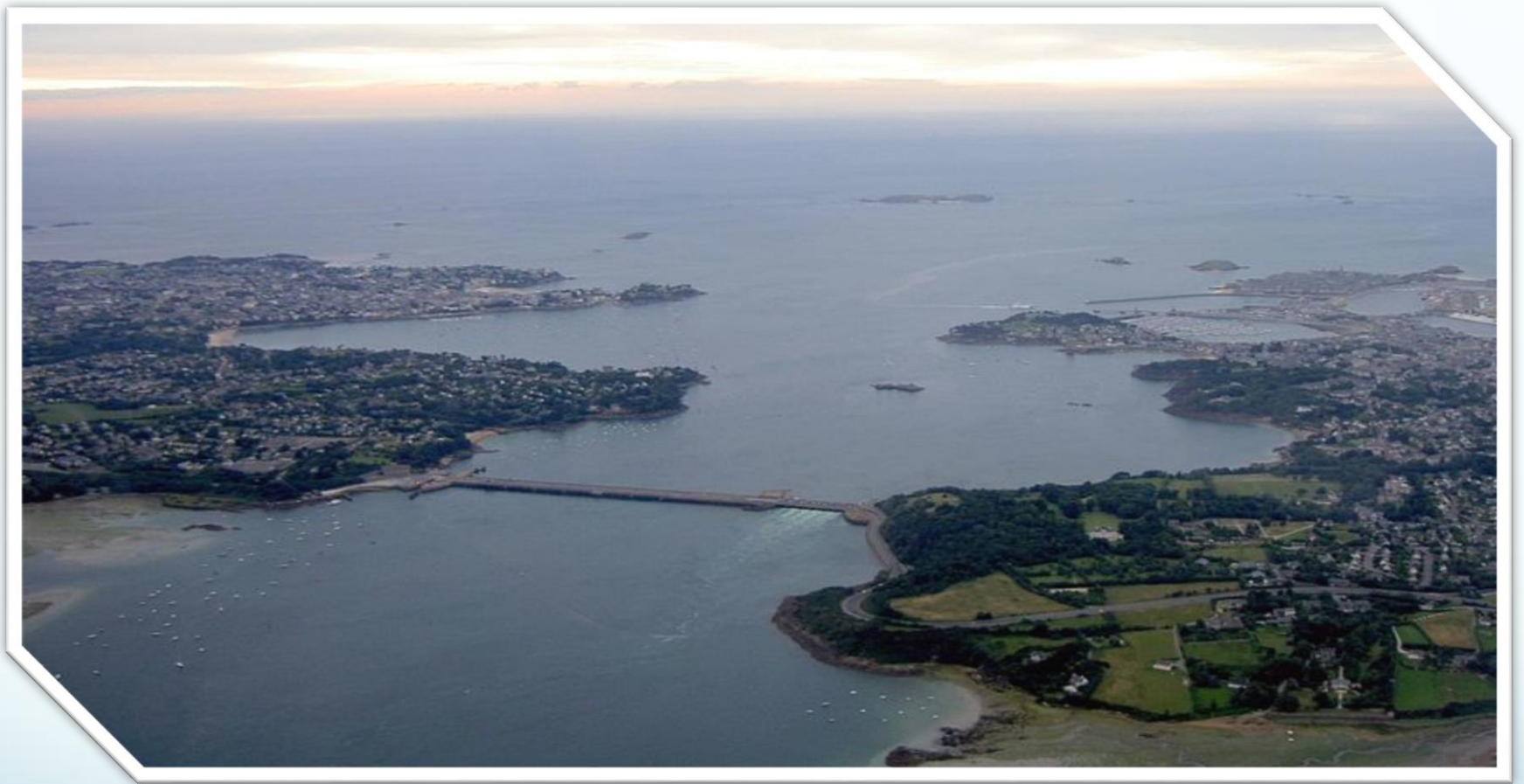
Rance Tidal Power Station, Brittany, France
