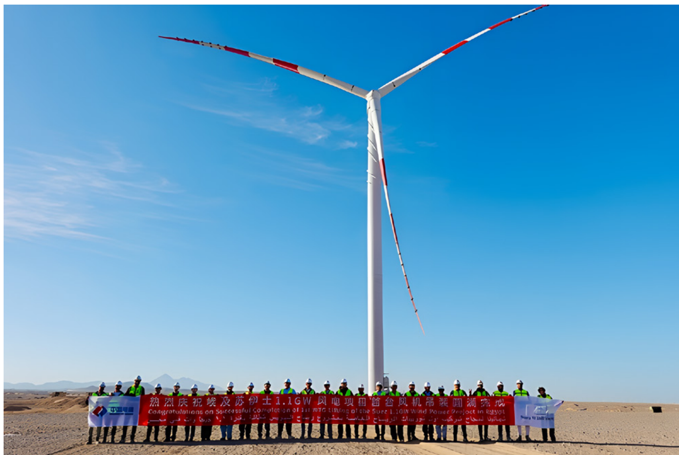
Figure 4-4: The first 8MW turbine installed in the 1.1 GW Gulf of Suez wind farm
