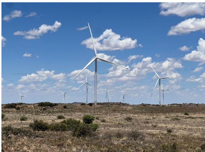
Photo: Courtesy of ACED
