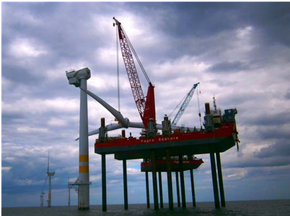
Figure 3.2. Example of jack-up platforms (Fugro Excilibur and Deep Diver) The jack-up platforms were used to conduct maintenance operations at the Arklow Bank Offshore Wind Farm, in the Irish Sea (Source: www.fugro.com )
