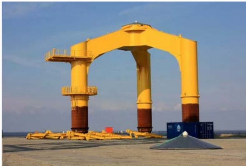
Figure 1.10. Tri-pile foundation used in BARD Offshore 1 wind farm
