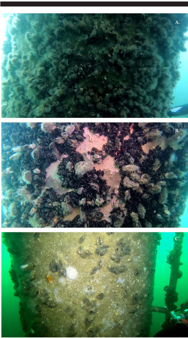
Figure 7. Representative images from video transects for Turbines 1 (top), 3 (middle), and 5 (bottom) all at midwater depth, showing simultaneous varying epifauna growth among turbine structures.
