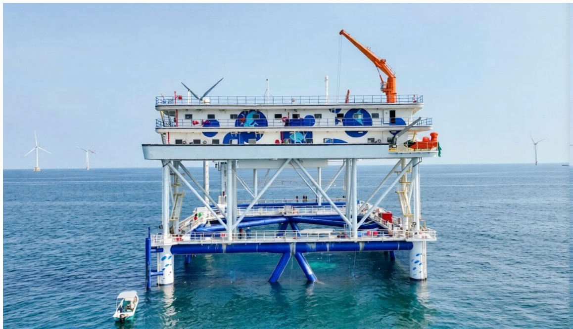
Figure 3. “Fuxi-1” ultra-large offshore wind–aquaculture integrated cage platform in Shanwei, Guangdong Province, China [14].
