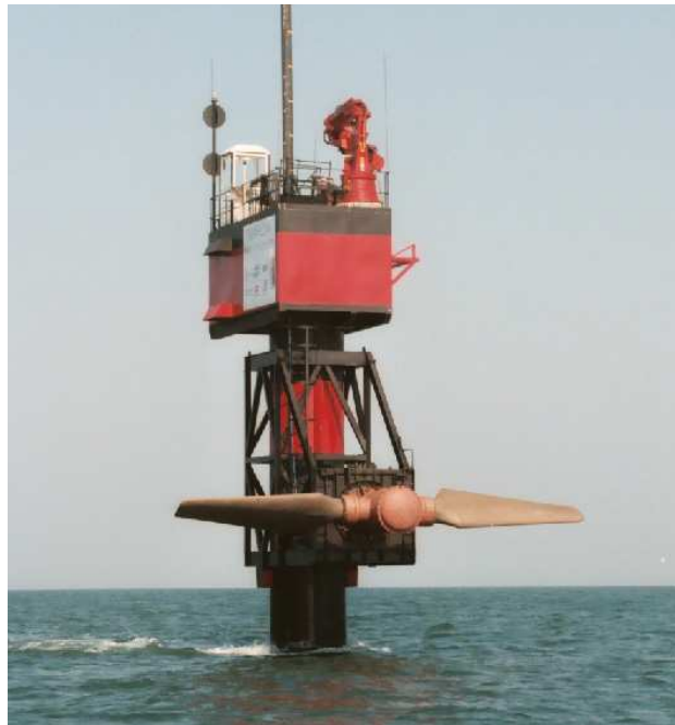
Figure 65 Seaflow installed off the north Devon coast in the Bristol Channel [89]
