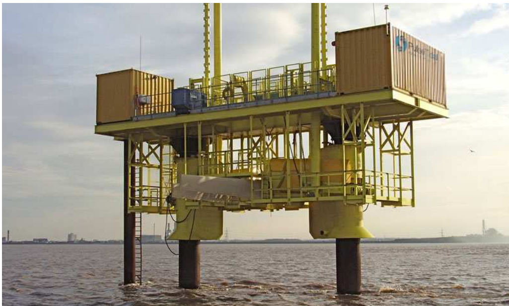
Figure 62 Pulse tidal device installed at the Humber estuary with the blades raised for maintenance [85]
