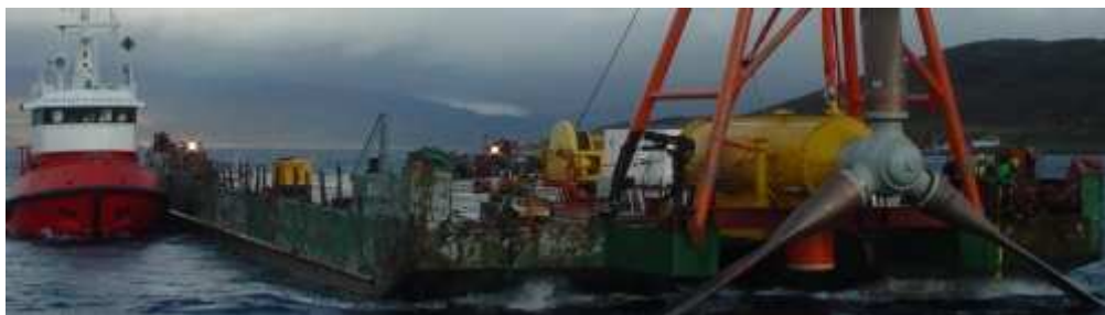
Figure 60 Hammerfest HS300 turbine during deployment at Kvalsund [81]
