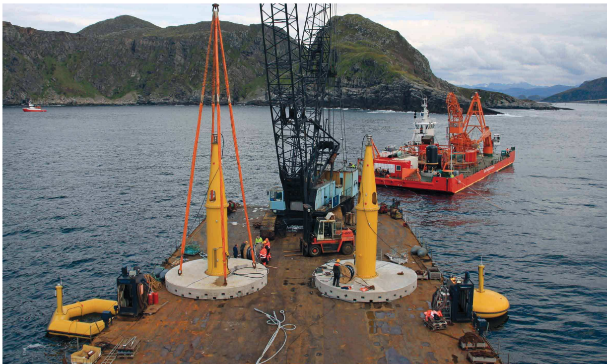
Figure 30 The two WECs being installed at the Runde test site, showing the buoys(in the water) together with the linear generator and gravity foundation (on the barge) [40].
