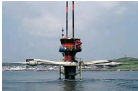
Full Scale (1.2MW) SeaGen prototype at Strangford Lough, Ireland (Photo: Marine Current Turbine Ltd)
