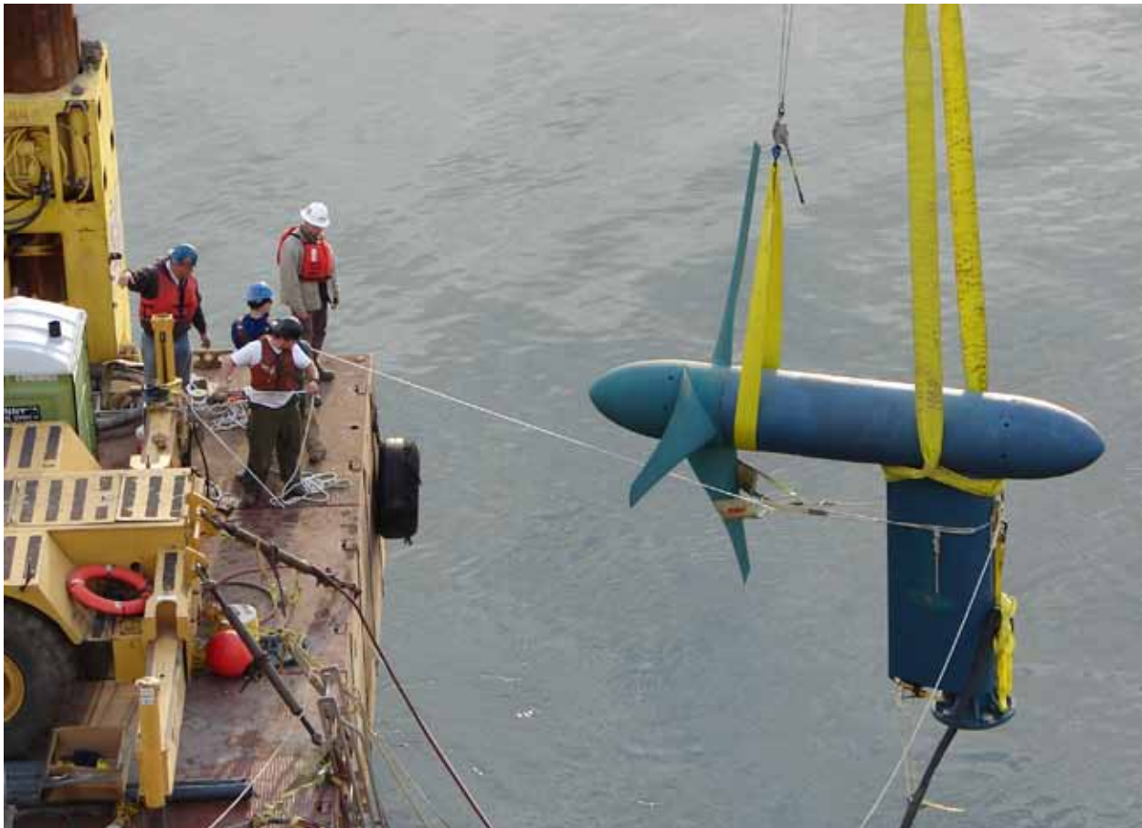
Figure 9 – Free Flow Kinetic Hydropower System (Source: Verdant Power)
