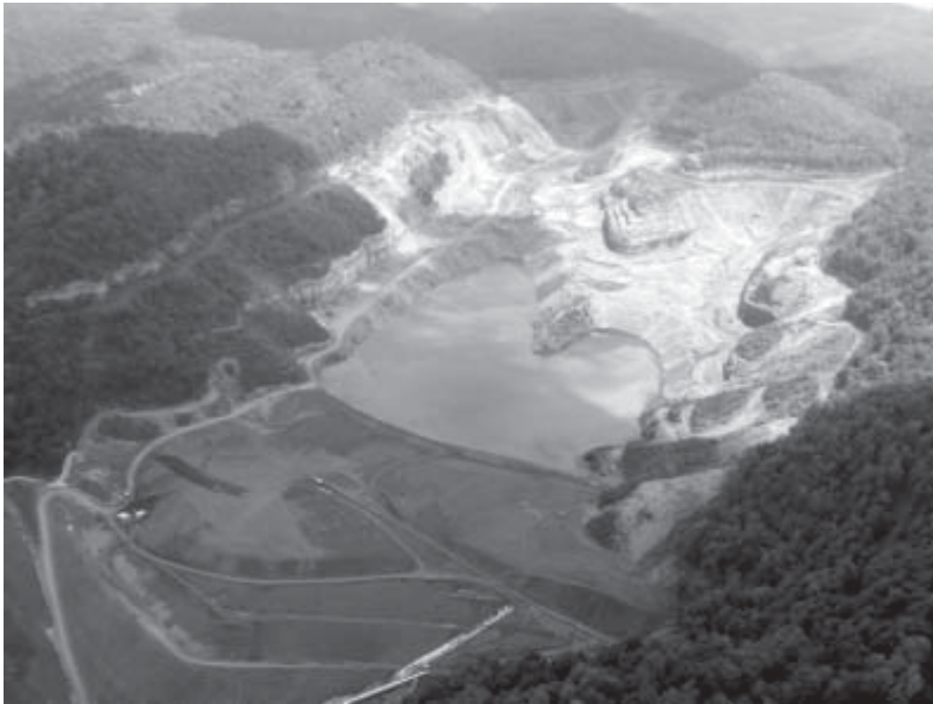
Marfork Coal's Brushy Fork coal slurry impoundment, which, at its final stage, will hold 8 billions of gallon of coal waste sludge. The impoundment partially lies over old underground mines and is directly upstream from the town of Whitesville, WV.
