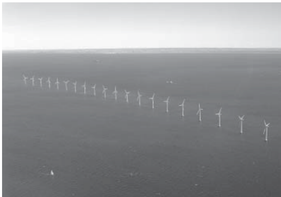
20 turbines, rated at 2 MW each, in Denmark's Middelgrunden Offshore Wind Farm.
