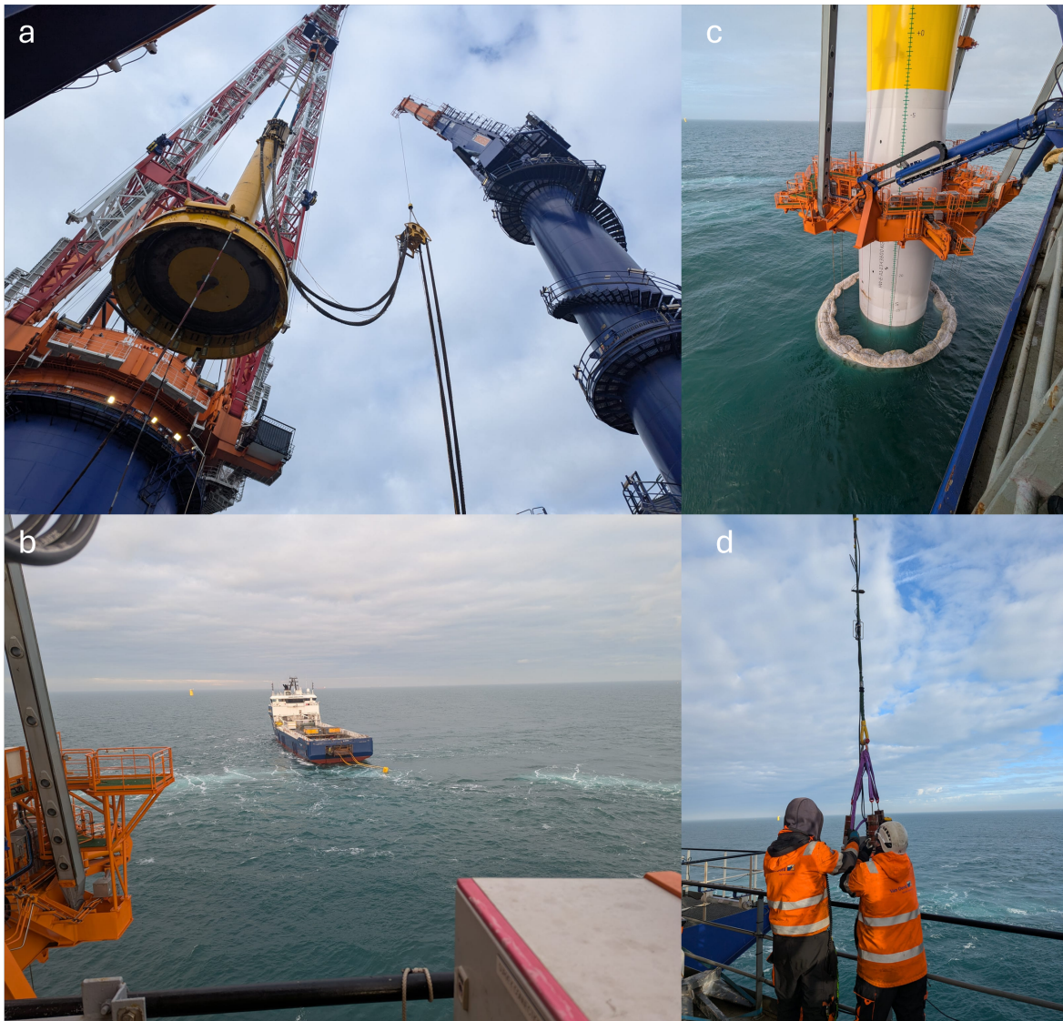
Figure 1.1: Impression of monopile installation works and measurement campaign, pictures taken from the Boreas. a) The impact hammer ready to be installed on top of the pile. b) The noise mitigation vessel with the bubble curtain active. c) The pile in the gripper with the HSD-net deployed and the dBBC in the background. d) Installation of the near-pile monitoring setup from the Boreas.
