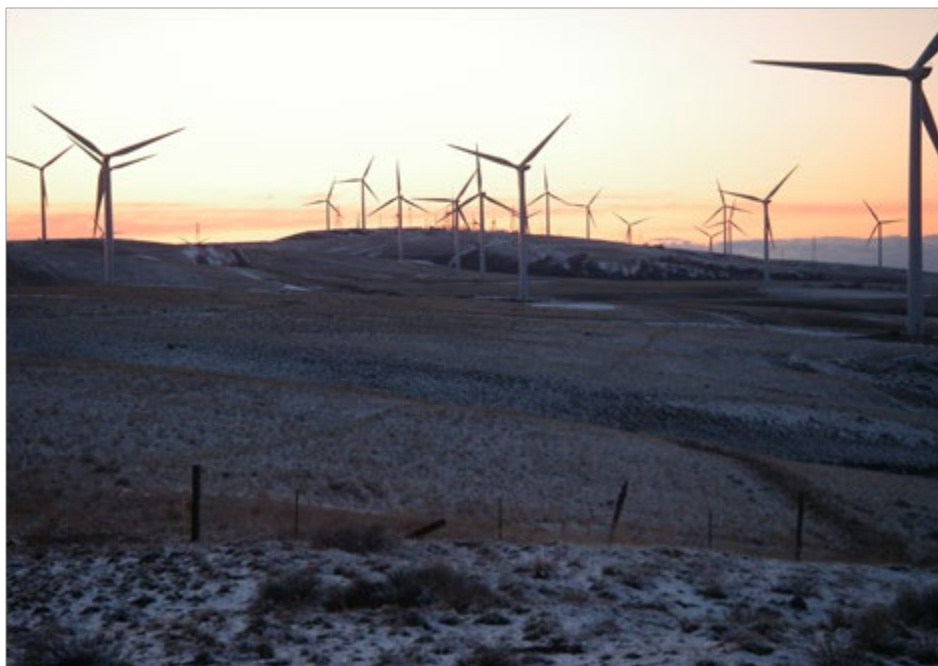
©Image from Rocky Mountain Power, a division of PacifiCorp.
