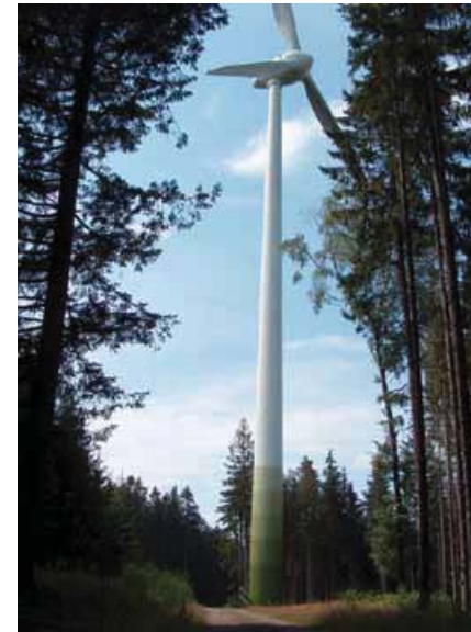
The setting of wind turbines in woodlands is highly dangerous for bats and therefore not recommended and criticized by the present guidelines. © H. Schauer-Weissahn & R. Brinkmann
