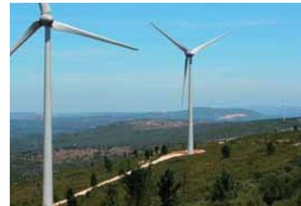
In Portugal, this 7-turbine wind farm has one located 158 m from an important hibernating roost (around 4000 Miniopterus schreibersii and 150 Rhinolophus ferrumequinum ). The cut-in speed of that turbine is increased to 5 m/s in October, November, December, March and April. © J. Rydell
