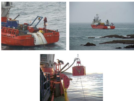
Figure 2. Details of submarine cable installation (above) and burial machine (below).
