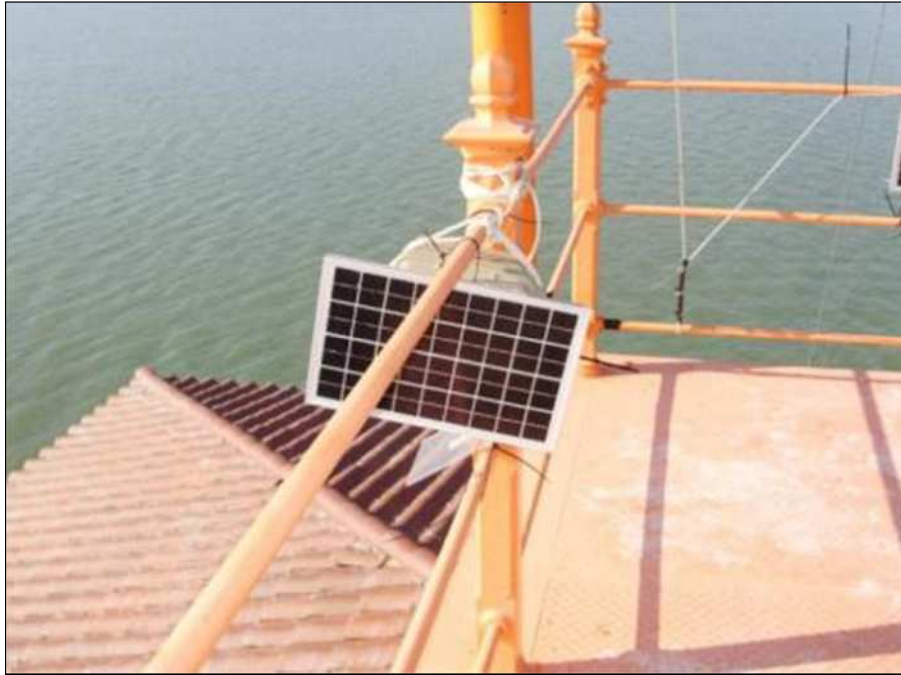
Figure D.3 West Rail detector on Crib, 2010
