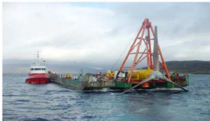
Figure 6: Installation of Nacelle
