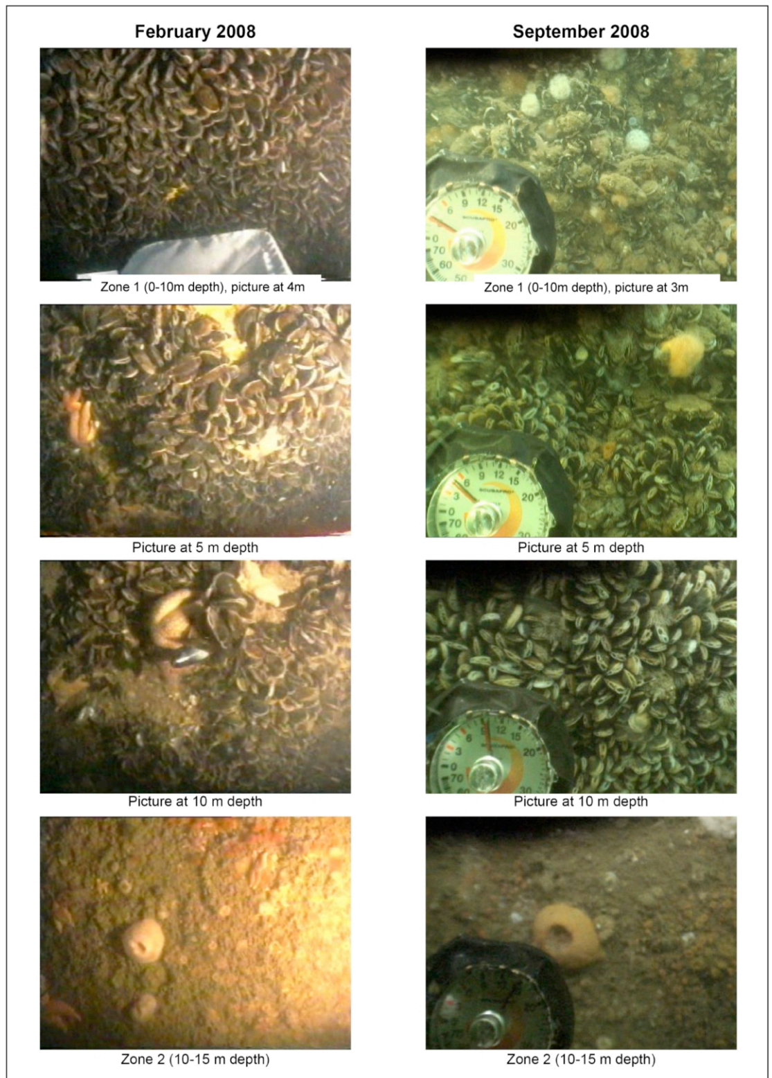
Figure 6 Underwater growth on the monopile of turbine 34 at different depths in February and September 2008.
