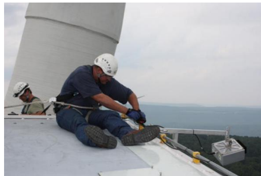
Figure 4. Attaching devices to a safety rail on the top of the turbine nacelle (Photo by M. Baker)
